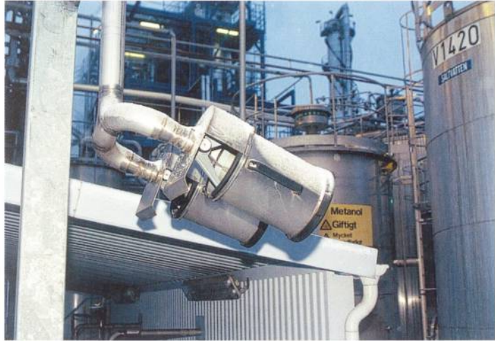
3.29 Fixed installation for medium-expansion foam.
