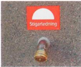
2.46 A rising main in a tall stairwell means that hoses do not have to be laid out. The inlet has a warning sign and is usually located behind a locked cover.
